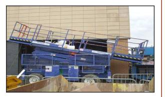
Fortunately the working platform had been raised less than 2 meters at the time and although the operatives were pitched forward, they were not seriously hurt and were able to climb down to ground level. The rear end of the scissor packs' scissor arms had sheared from their base pivot—pin connectors as shown below, the close up shows one of these two failures.
